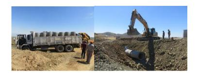
Figure 4. Concrete pipe culverts
